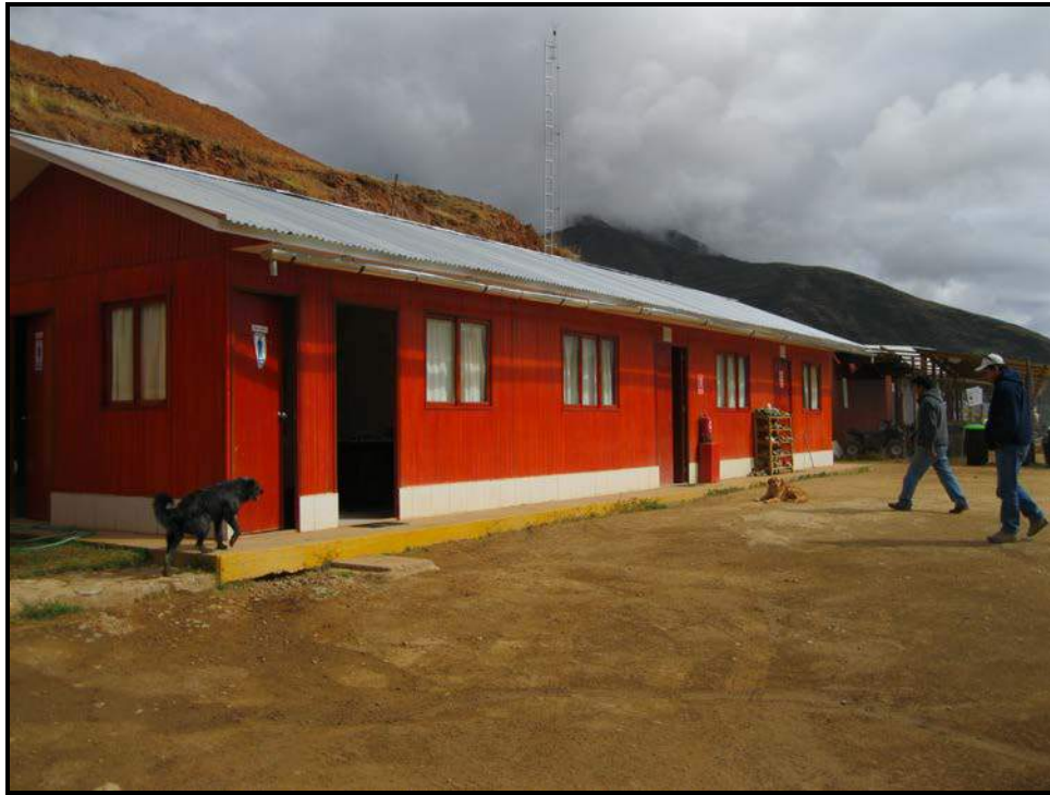
Figure 12.5 Cotabambas Base Camp
